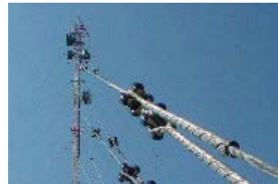
Guy Wire Insulators
