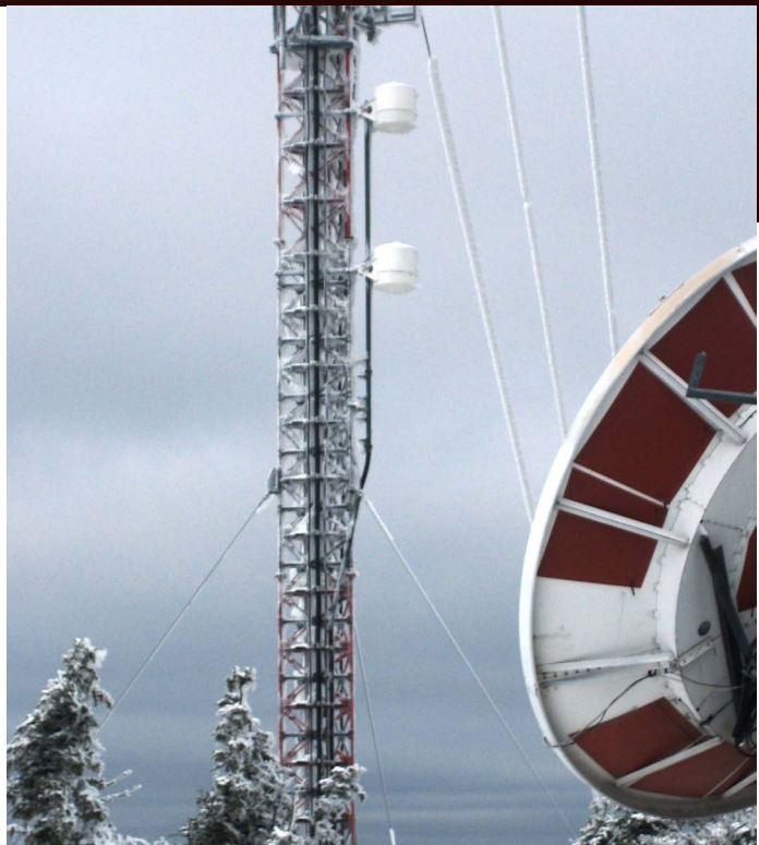
Directional FM antenna systems raise some particular questions. Shown is a Dielectric DCR-H system with radomes.
