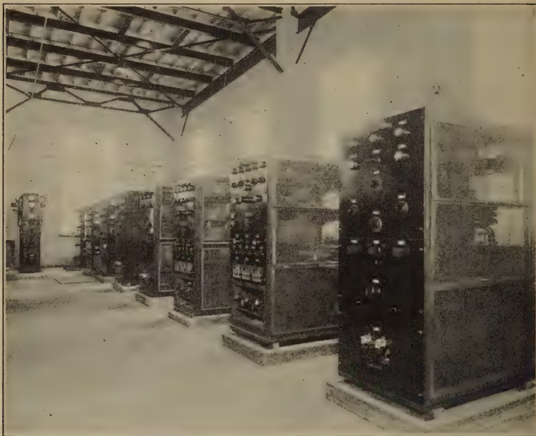
FIG. 270. A Group of High Frequency Transmitters Operated by the Radio Corporation of America at Rocky Point, L. I.
