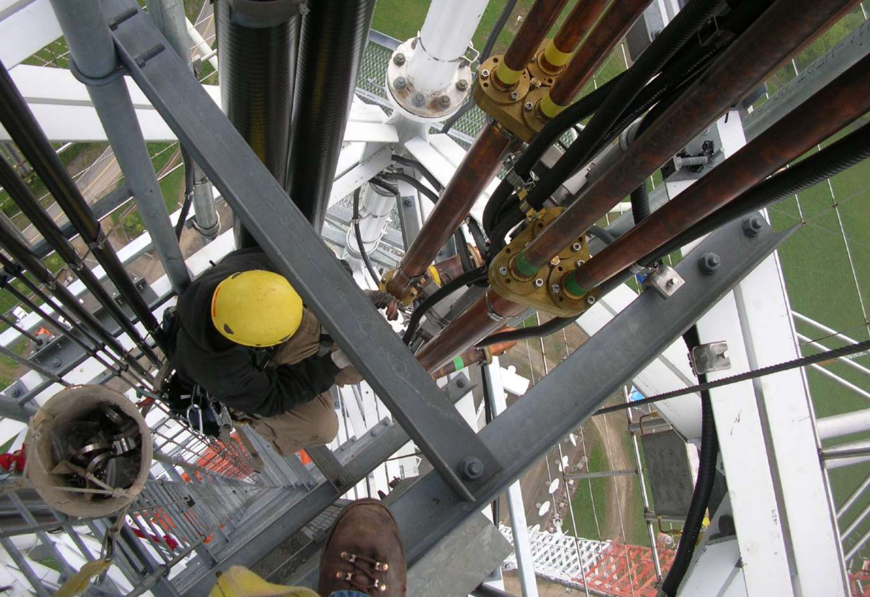
Above: Installation of coax hangers.
