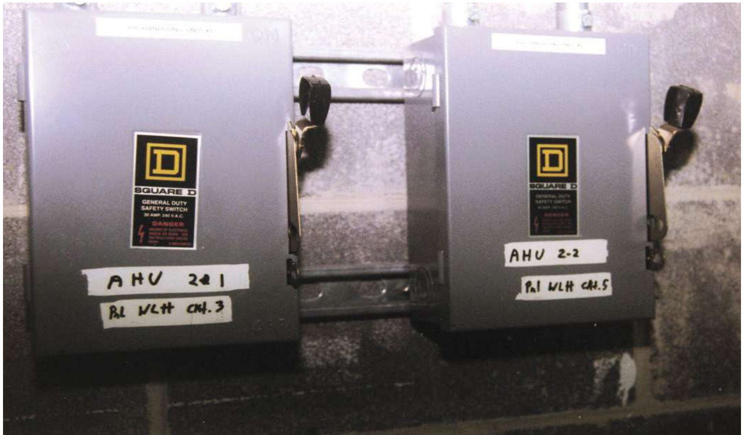
Above Fig. 12: Duct or gaffer’s tape works just fine for identifying AC disconnects.
