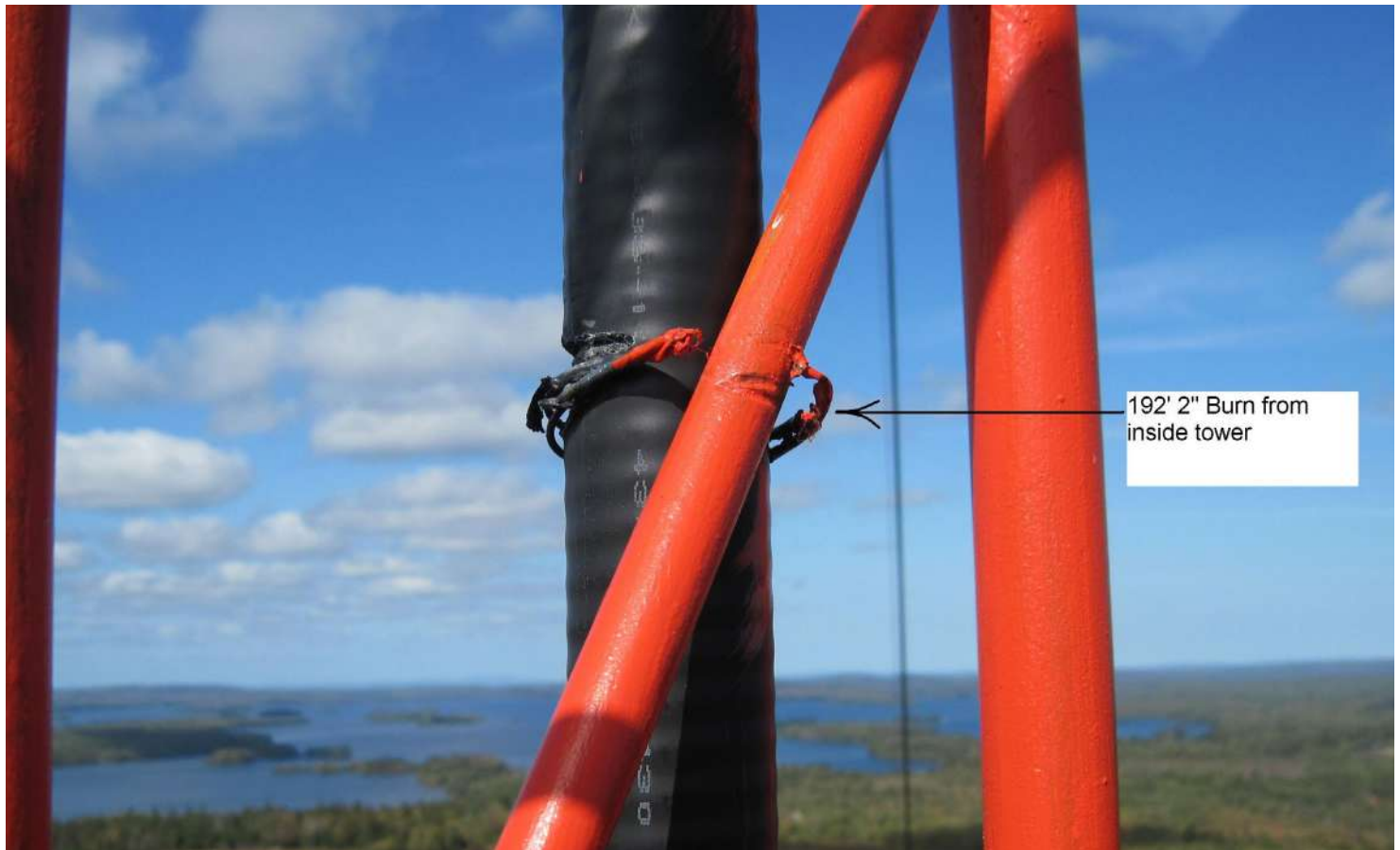
Above Burns are visible where wire had been used to secure a flexible 3-inch line.
