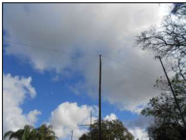
Helically wound vertical with wire top loading
