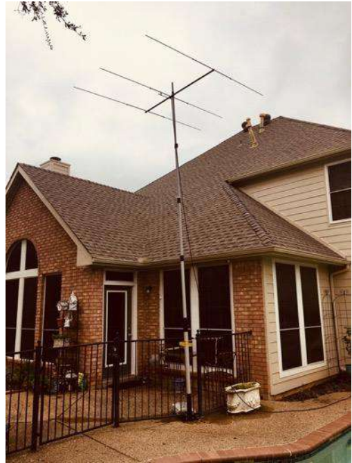
Figure 22 - M2 3-element Yagi
